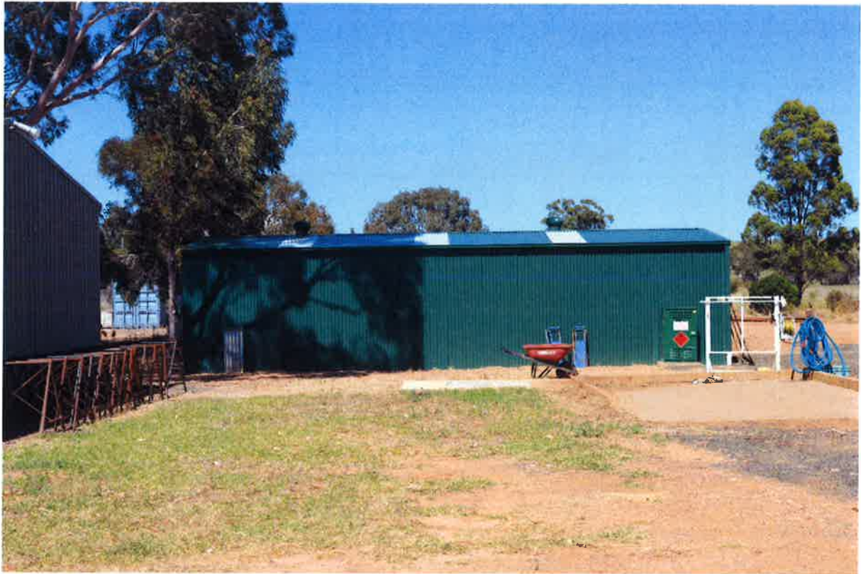
Photo 13: Maintenance shed erected on the slab of the former Aminya laboratory that serviced the mining operation 1996-2002. Photo taken 29 November 2022.
