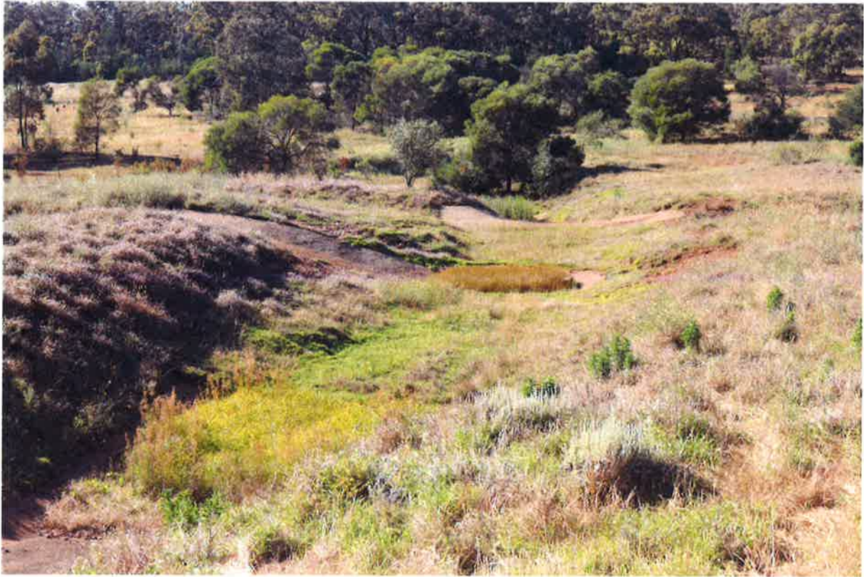
Plate 21. The downslope flumes constructed on the WRE in 2002 by Soil Conservation service are working effectively. This image taken 29 November 2022 shows three stilling ponds each supporting a dominant wetland species ( Cyperus sp. , Juncus sp. and Typha orientalis ).
