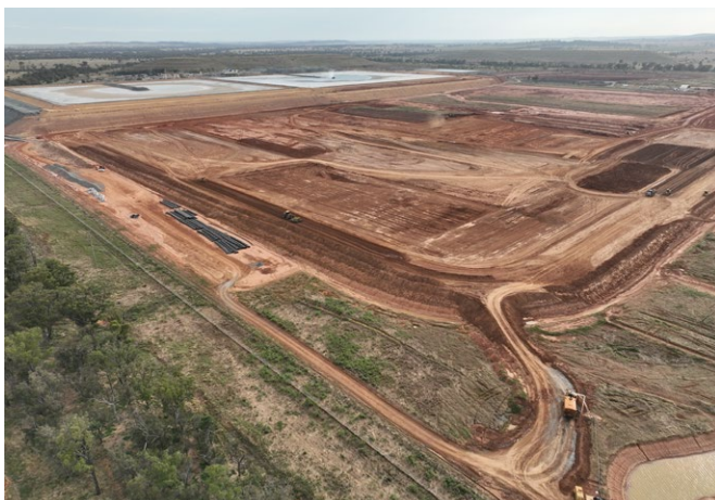
RSF2 under construction
