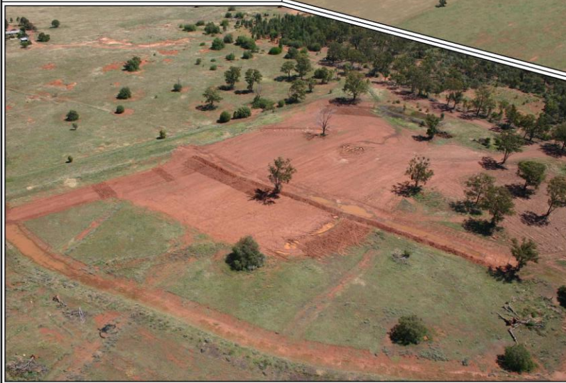
Plate 3: Top Soil Stockpile Area Recontoured. (Ref: 4 Dec 2005)
