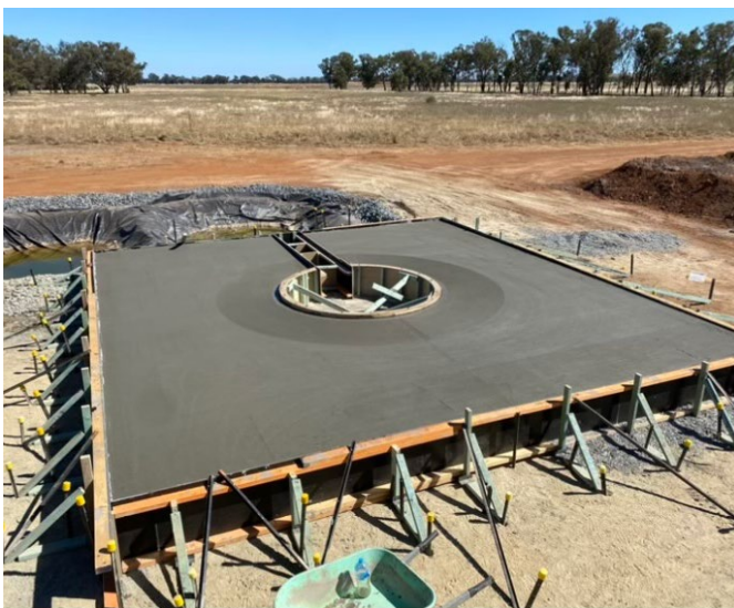
Construction of the cap for the vent shaft
