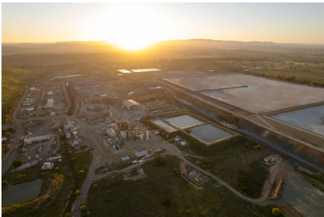
We're seeking approval for a final wall lift on RSF1
