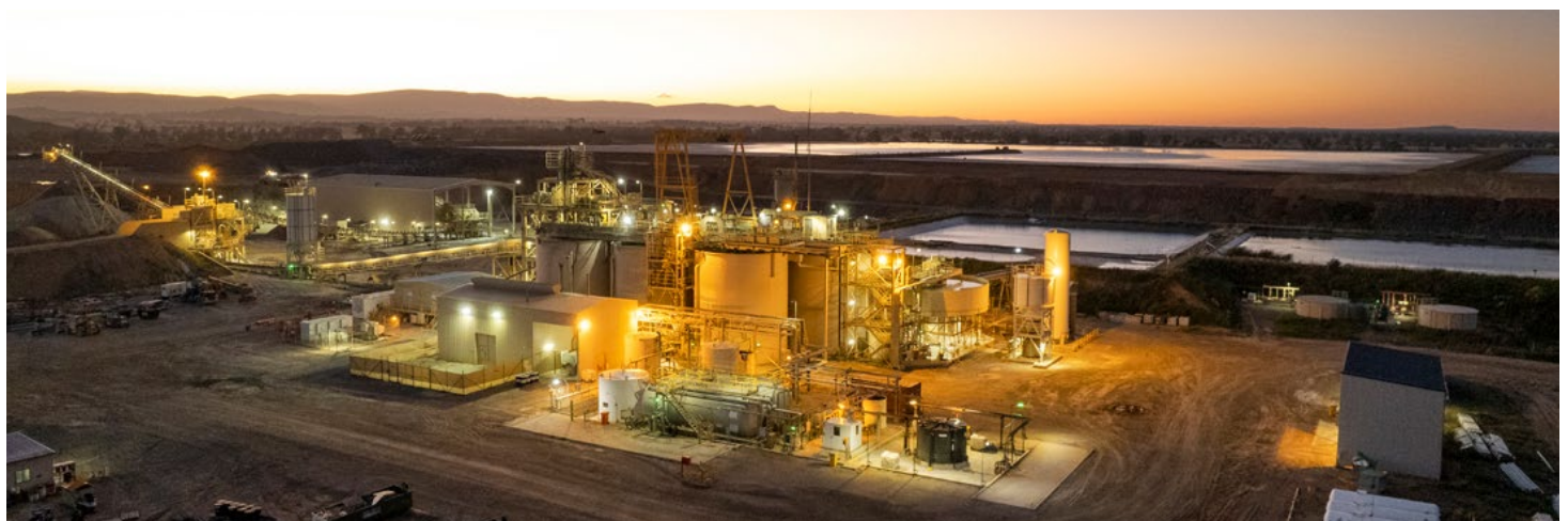
The Tomingley Gold Extension Project will extend the life of the TGO processing plant.
