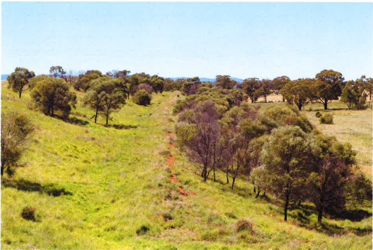
Photo 14: Heap leach berm looking south. Currawang ( Acacia doratoxylon ) grows on the west facing batters.
