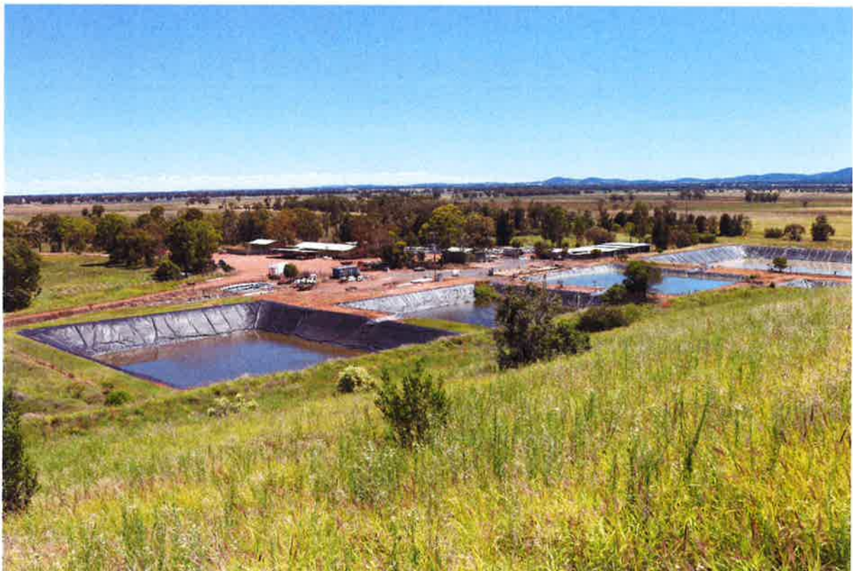
Photo 10: View of HDPE-lined ponds, core yard, office and house at Peak Hill Gold Mine.
