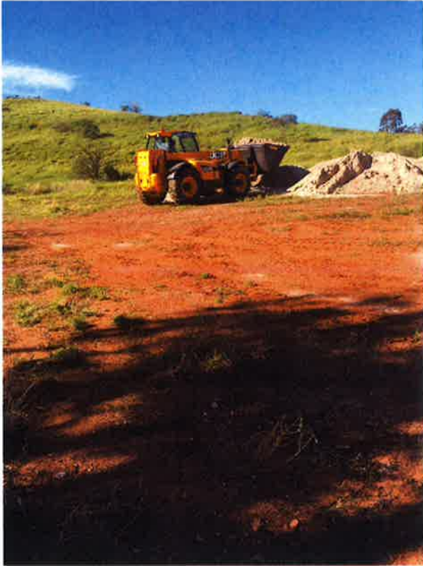
Photo 19: Agricultural lime for final landform top dressing April 2021. Photo by Ken Robinson.
