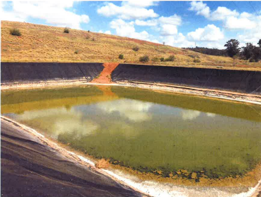
Pregnant overflow pond. The PHGM processing ponds remain to be rehabilitated in MOP 2014-2022.
