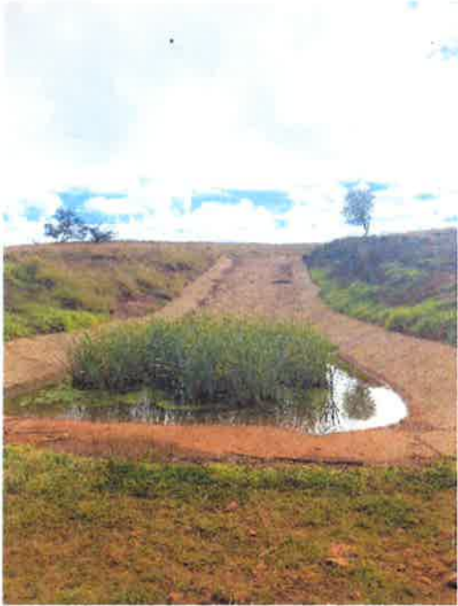
PHGM WRE flume designed and constructed by NSW Soil Conservation Service in 2002. Photo taken 31 July 2020
