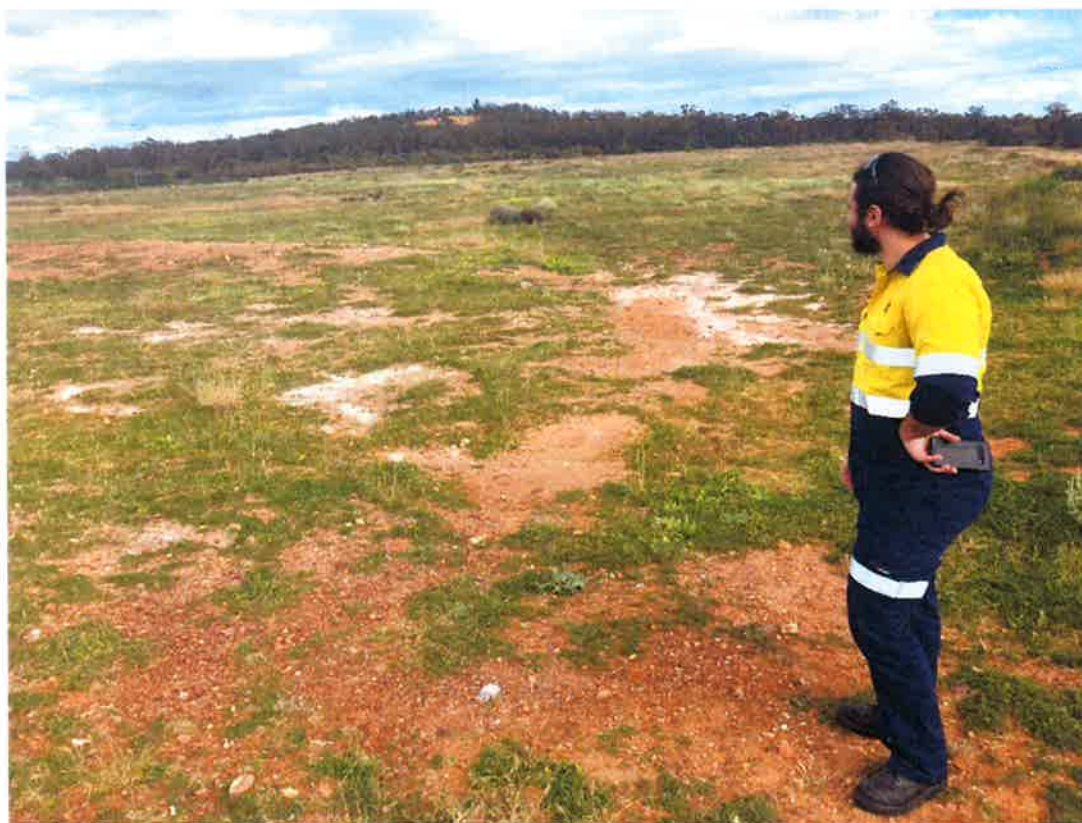
Resources Regulator inspecting localised salt sweats on heap leach final landform 19 June 2020. Ag lime to be spread March 2021 should partly remedy this phenomenon.
