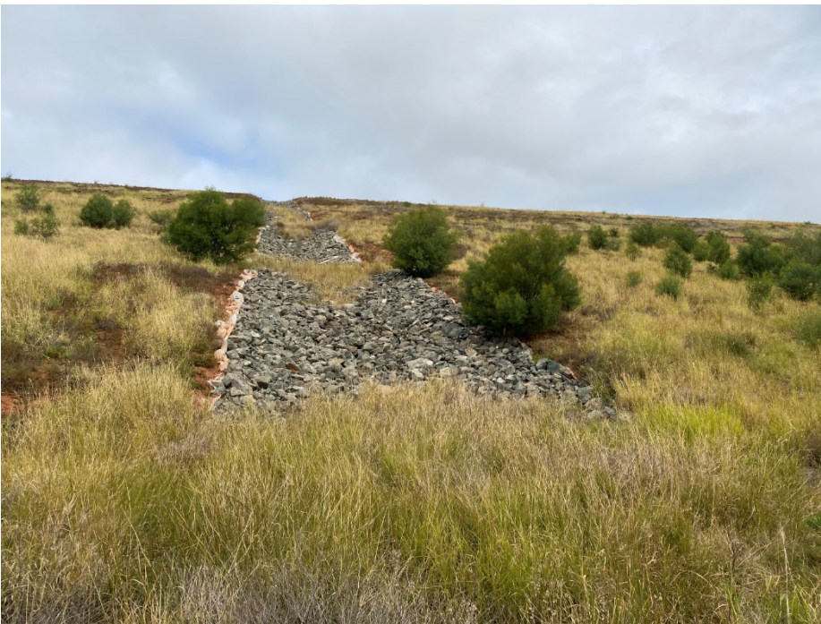
Photo 2 - Established rehabilitation and stable drop structure
