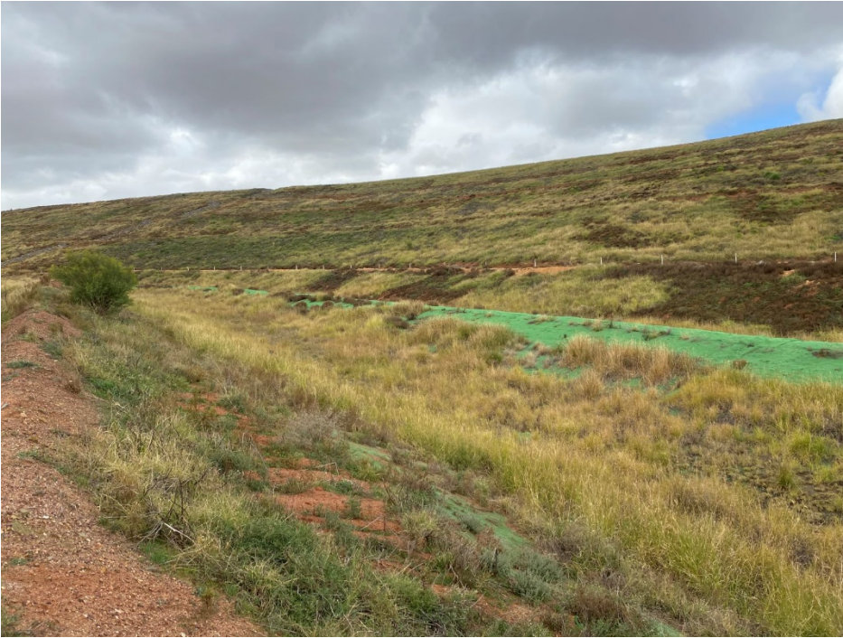
Photo 5 – Stable drain and rehabilitation area
