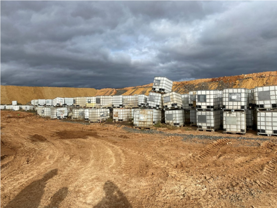
Photo 9 – Empty hydrocarbon storage that are not stored within bunds
