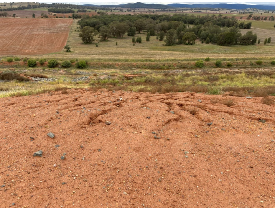
Photo 6 – Some areas of erosion in sections of rehabilitation
