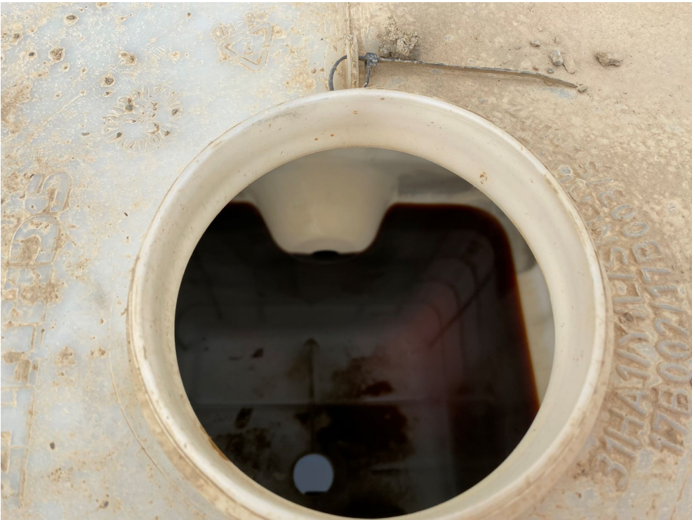
Photo 9 – Empty hydrocarbon storage that are not stored within bunds
