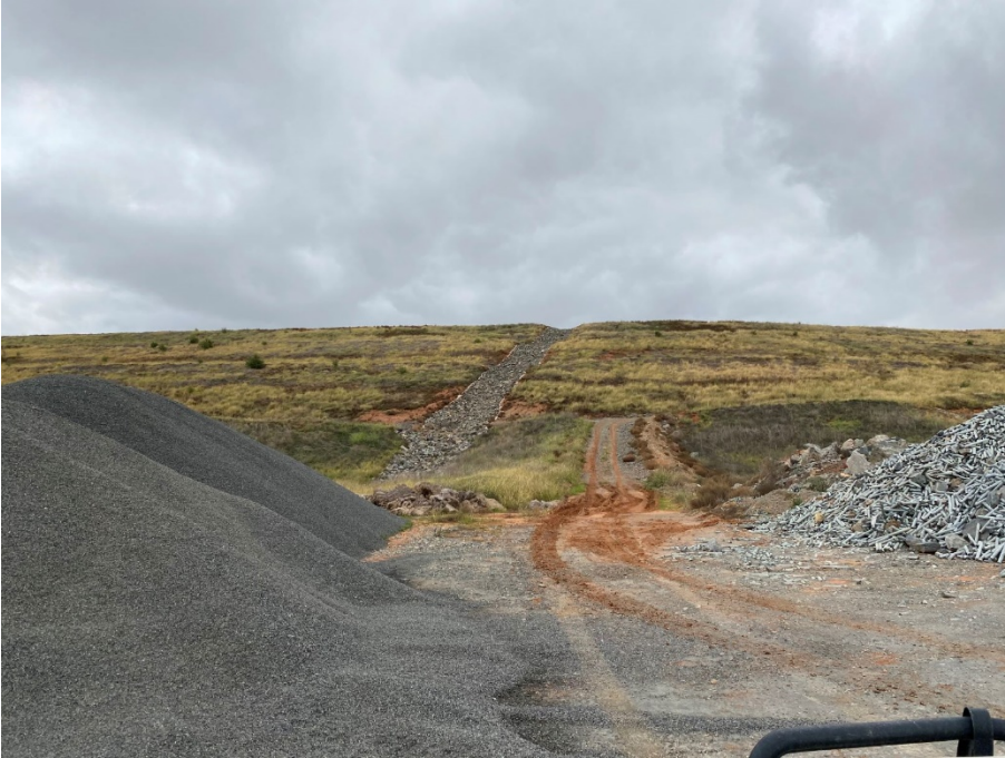
Photo 1 – Established rehabilitation and stable drop structure
