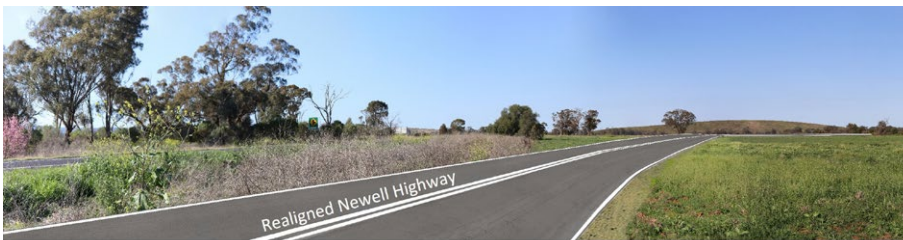
Highway Location 1: After mining
