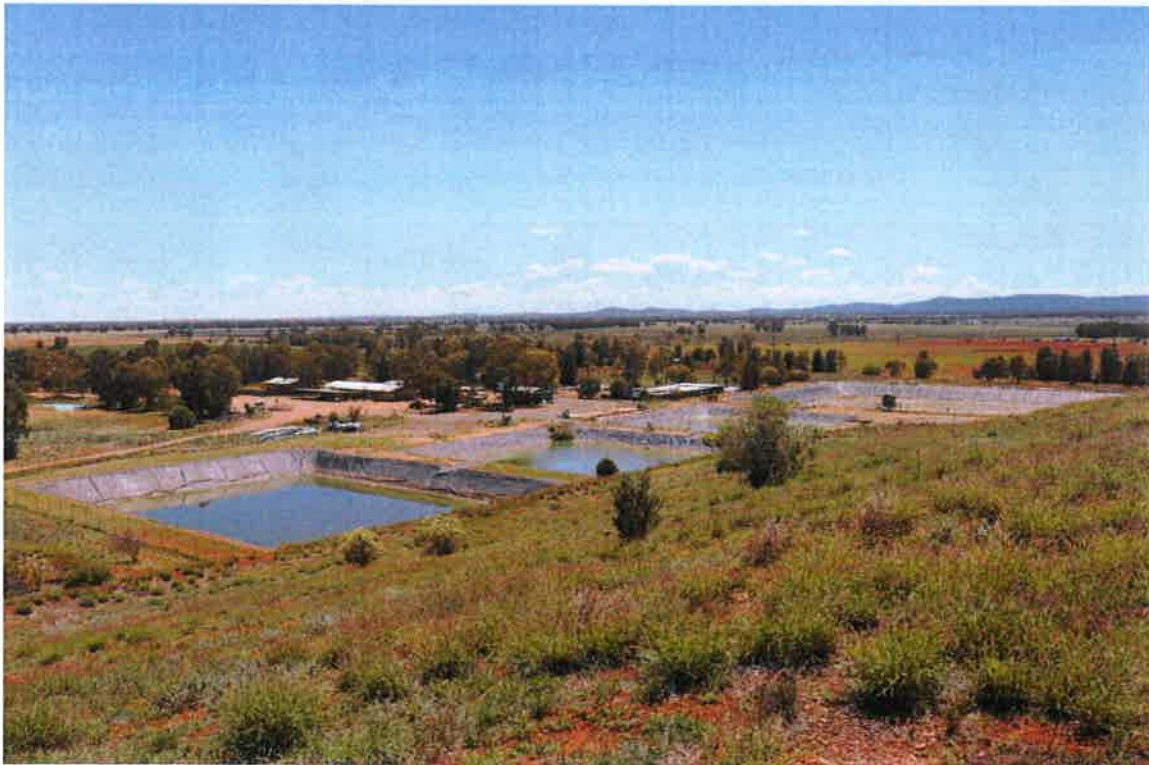
The remaining infrastructure at PHGM seen from the top of heap leach landform. Photo taken 17 December 2018.
