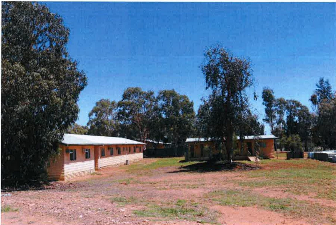
PHGM site office, crib hut and exploration house (background). Photo taken 17 December 2018.
