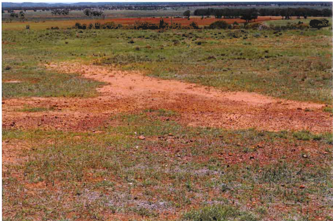
Small outbreaks of acid mine drainage and salt on heap Leach final landform will require lime and topsoil treatment. Photo taken 17 December 2018.
