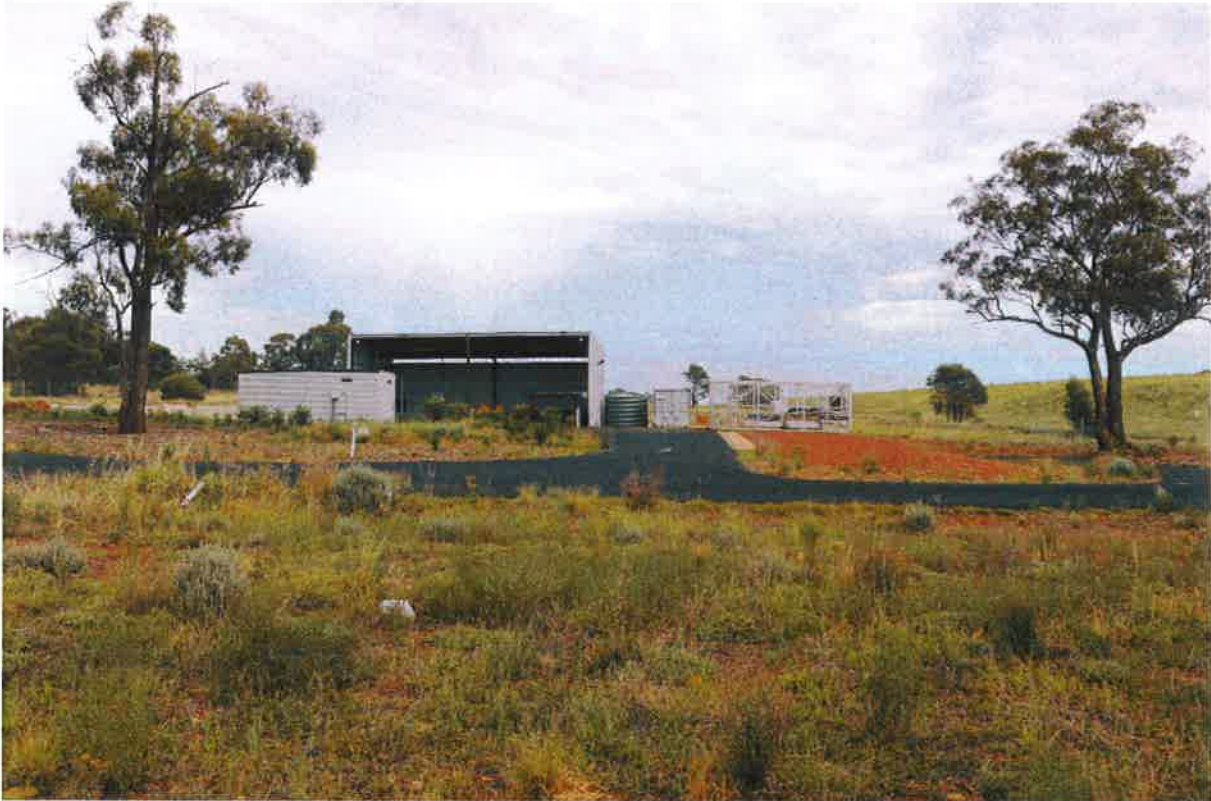
Parkes Shire Council Waste Transfer Station (not yet open for operations). This development is situated on 4 Hectares of land excised from the Mining Lease and gifted to Parkes Council by Alkane Resources Ltd in fulfilment of a consent condition Ltd. Photo taken 17 December 2017.
