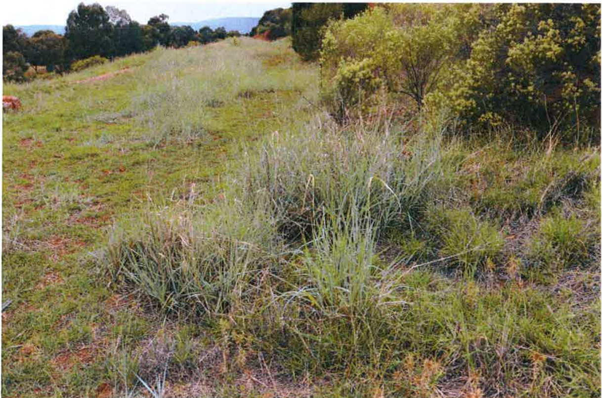
Premier digit grass and natural regeneration of Cassinia on upper batter of the WRE. Photo taken 17 December 2017.
