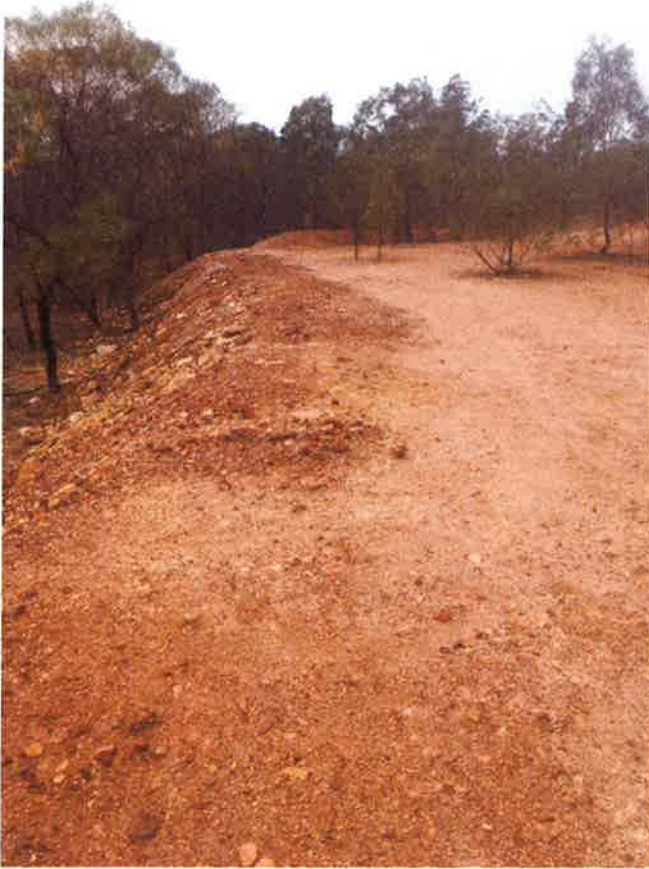
Haul Road to Proprietary pit with sulphide contaminated windrow removed to the toe of Gilligan's Island in July 2019.
