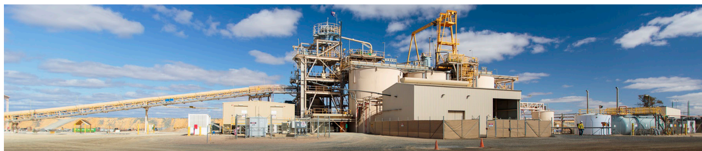
Tomingley Gold Operations plant
