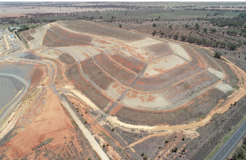
TGO has completed rehabilitation works on the WREs
