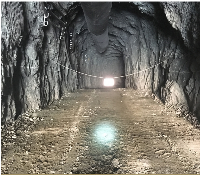
Photo of the underground decline
