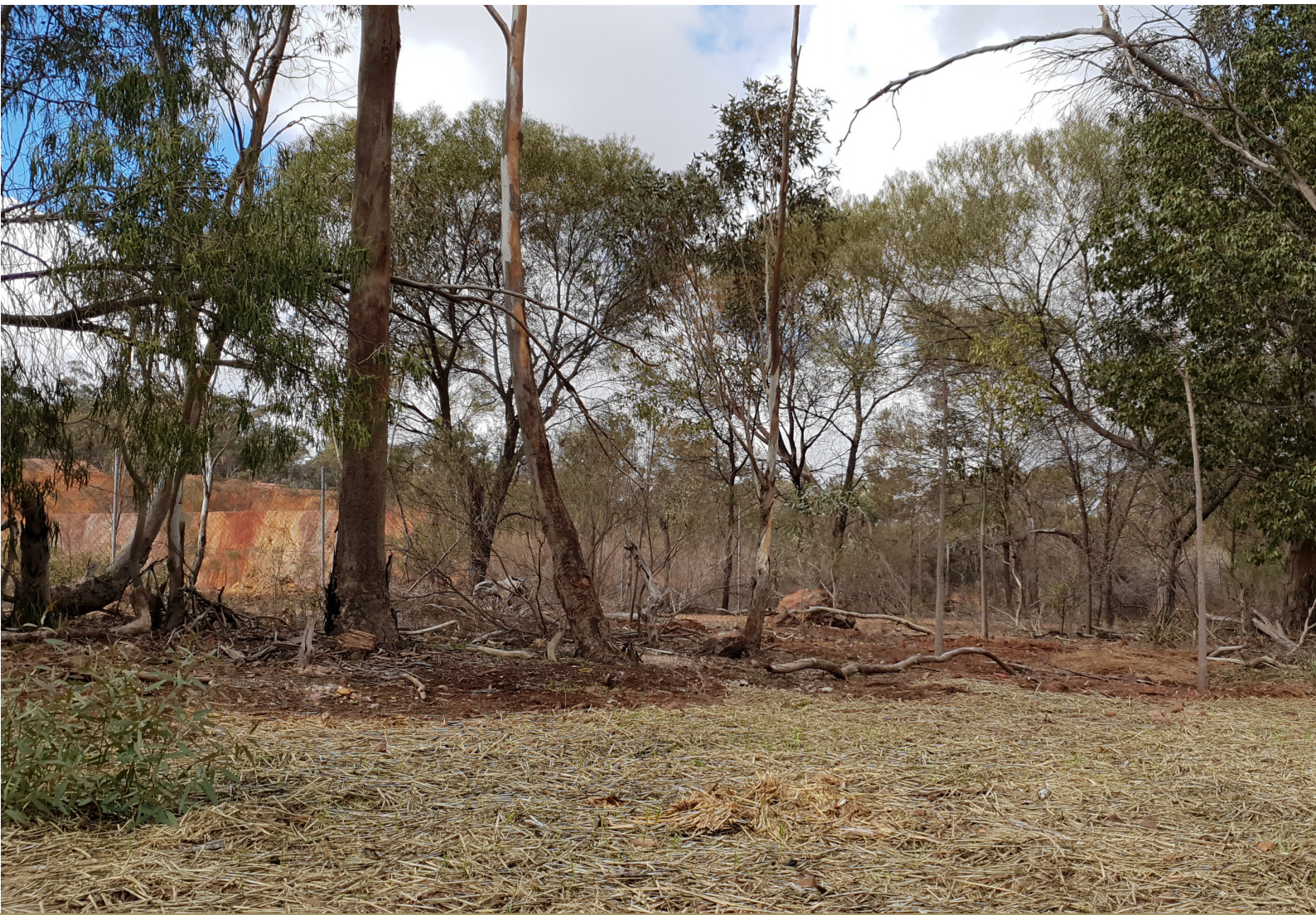
Newly transplanted native Currajong trees, which had to make way for drill rigs.
