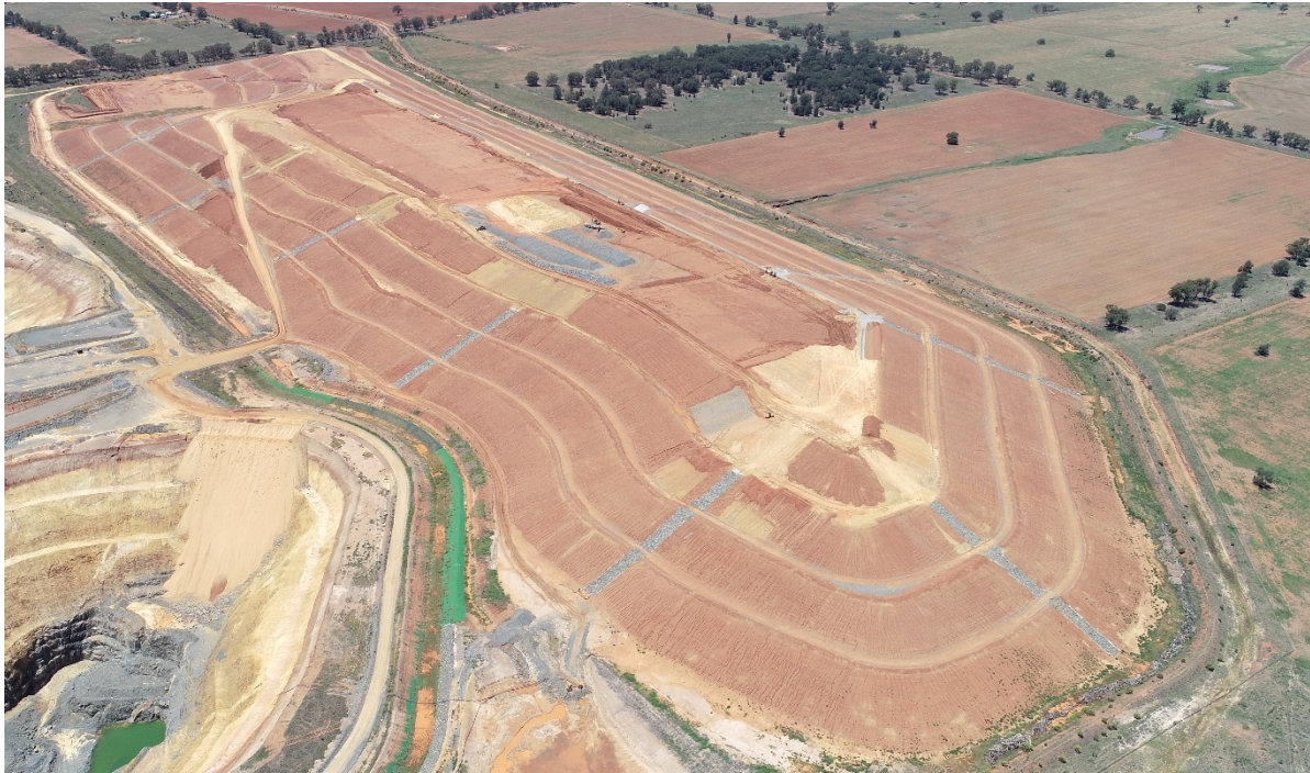
Plate 4: Reshaping and revegetation at WRE 3.
