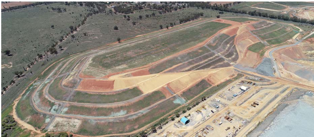
Plate 3: Reshaping and rehabilitation works at WRE 2.
