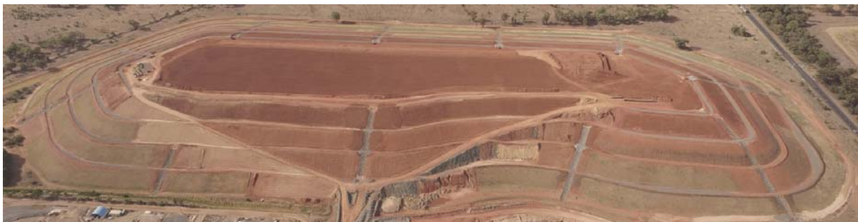
Plate 3: Reshaping and rehabilitation works at WRE 2.
