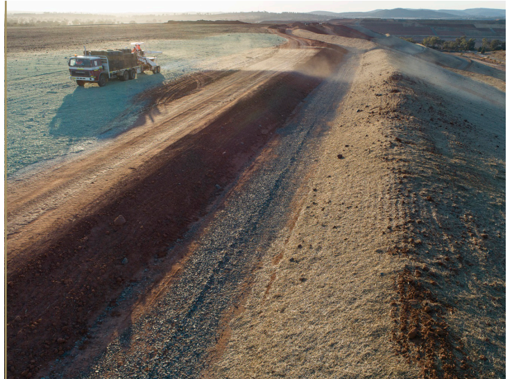
Rehabilitation of waste rock emplacements continues with seeding of vegetation
