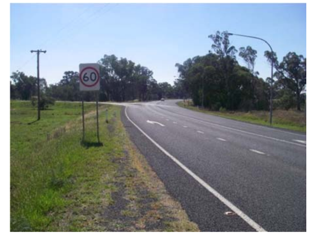
Photo 6. Intersection of Newell Highway and Narromine Road (Taken from the Newell Highway looking towards Narromine Road – 20/4/09)
