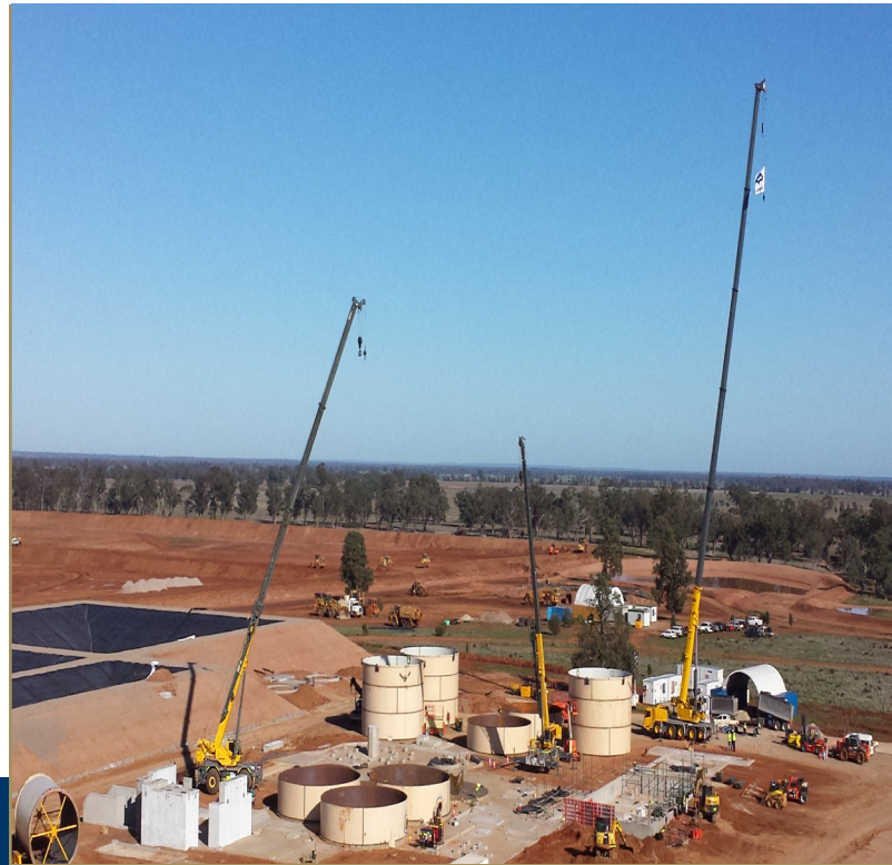
Aerial photo of the construction site
