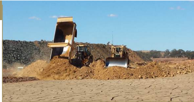
Works to lift the wall of the RSF
