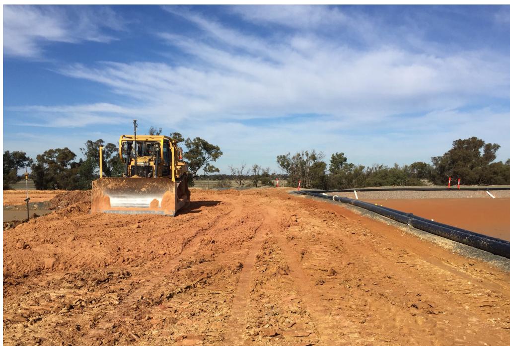
Works to lift the wall around TGO's residue storage facility
