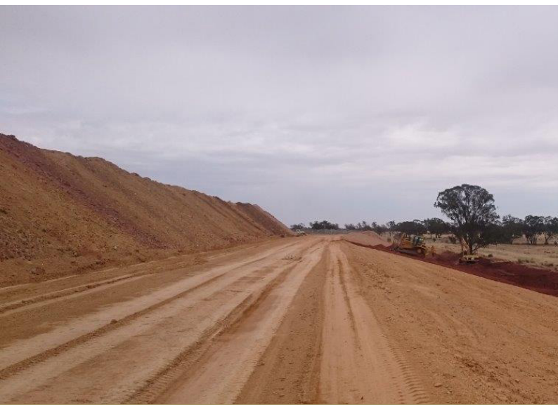
TGO has commenced rehabilitation of 'Waste Rock Emplacement Two'
