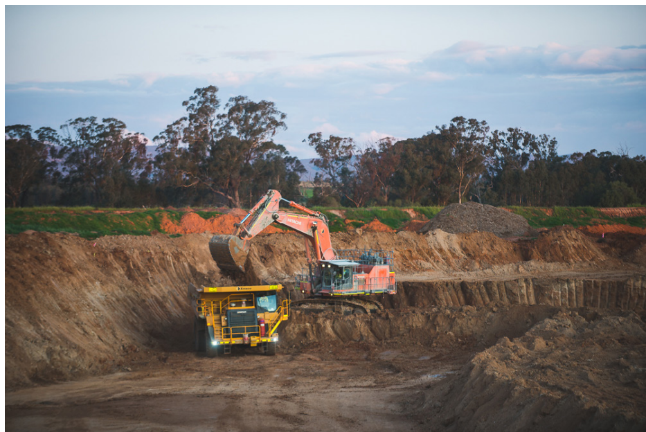
Operations underway at Wyoming One pit
