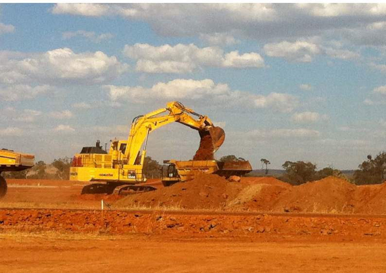
200t excavator loading a 777 dump truck with top soil
