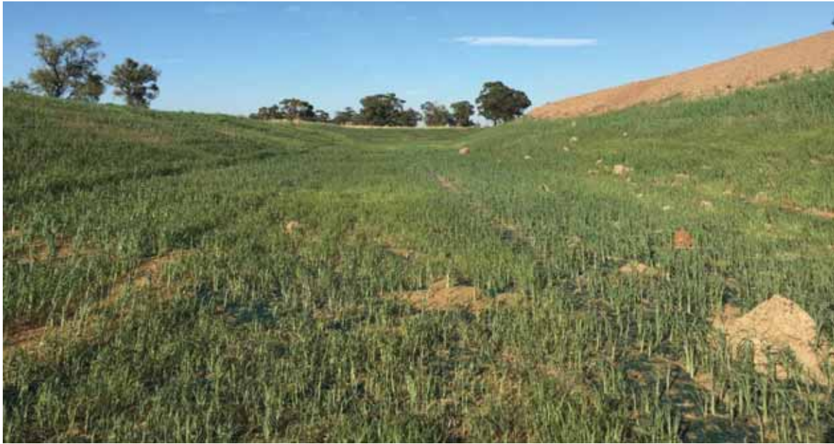
Plate 4: Revegetation following re-alignment of Caloma Central Drain.
