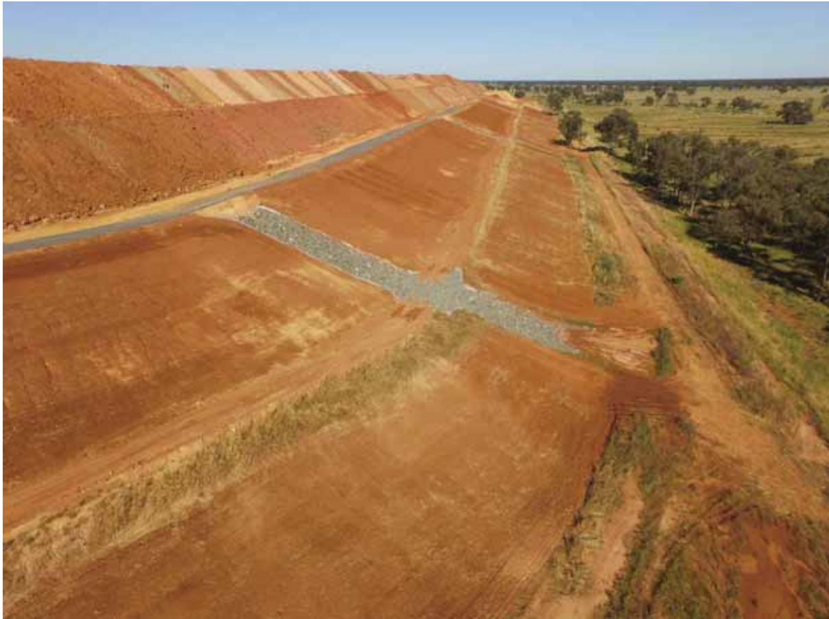
Plate 6: Reshaping works at WRE 2.
