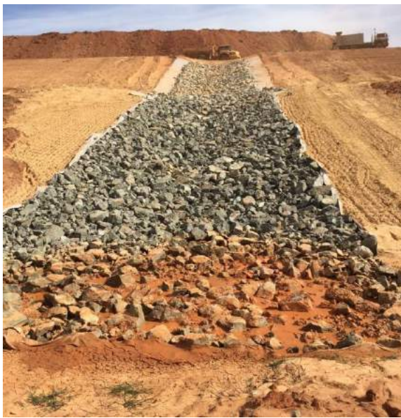
Plate 5: Drop structure construction at WRE 2.
