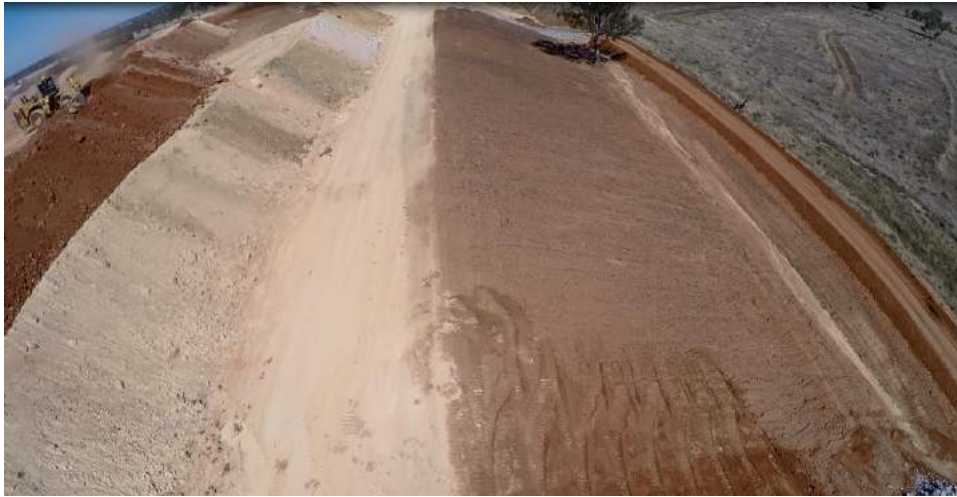
Plate 4: Reshaping works at WRE 2.
