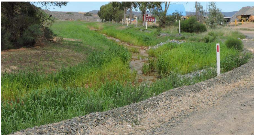
Plate 2: Dirty Water Drain January 2016
