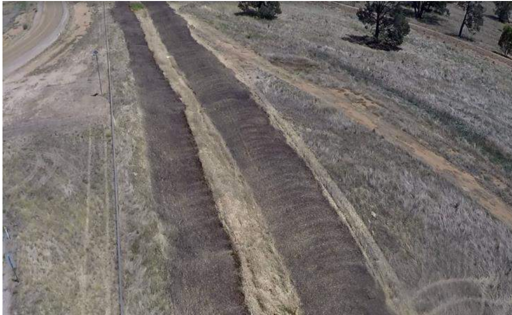
Plate 1: Dirty Water Drain immediately post rehabilitation (December 2015)
