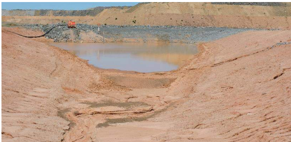
Plate 3: Enlargement of Sediment Basin 5
