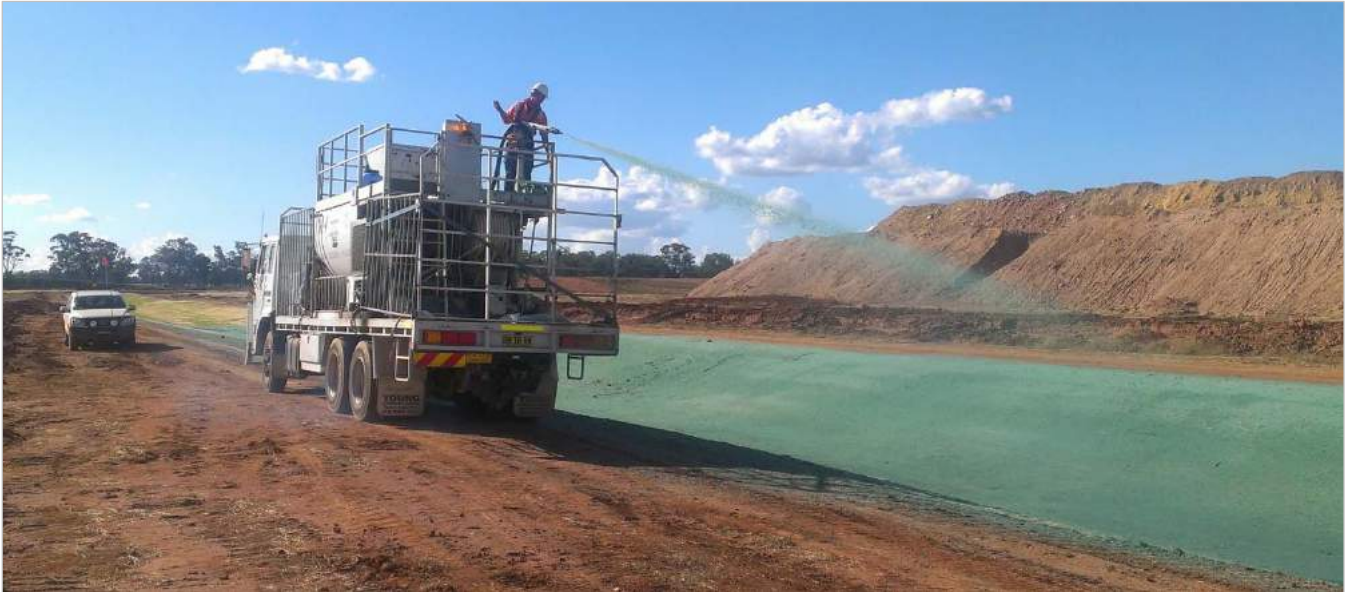
Figure 16: Hydroseeding of Caloma Drain
